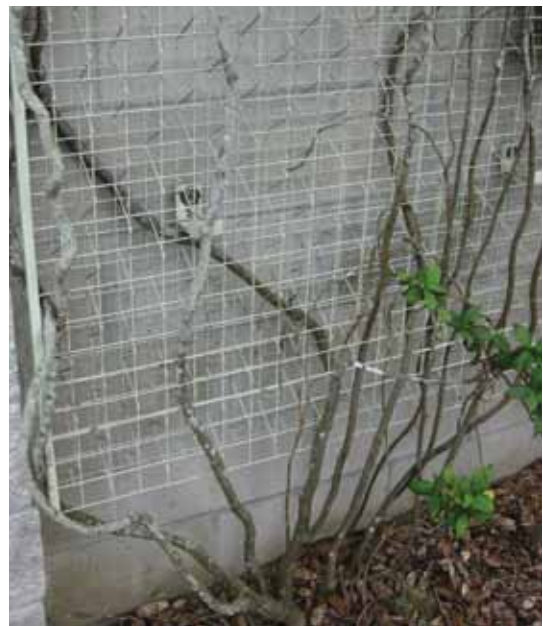
Figure 11. A trellis or other support should be placed several inches away from walls.
