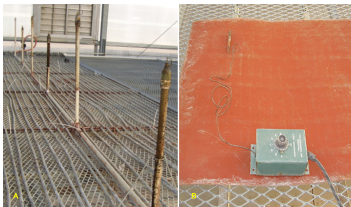
Figure 7. In this misting chamber for plant propagation, note that the tubes placed on the propagation bed carry hot water to provide bottom heat (A). Alternatively, heating pads can be used (B).
