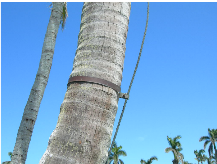
Figure 18. Close-up of the down cable that carries the current to the ground. Credits: A. D. Ali, The Davey Tree Expert Co.
