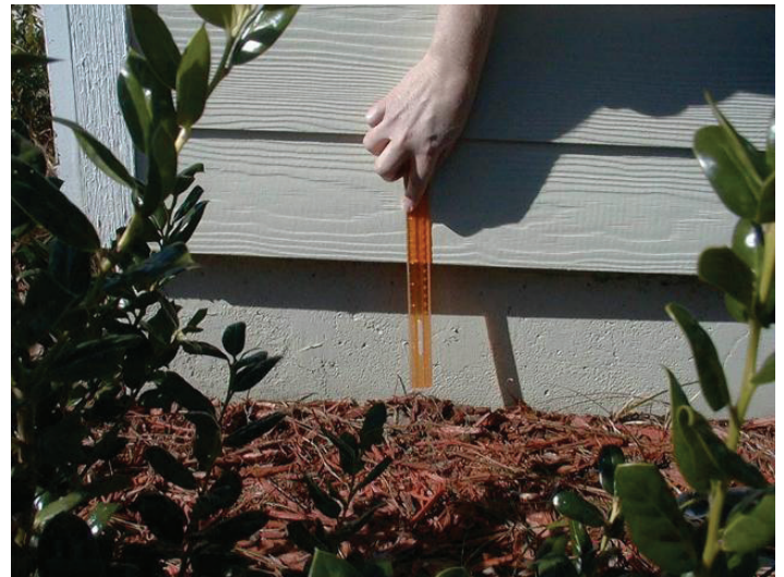
Figure 1. The building code requires at least a 6 inch inspection gap, as shown in the picture above. The inspection gap between mulch and siding on the home will allow anyone to see if termites are building mud tubes into a structure.
