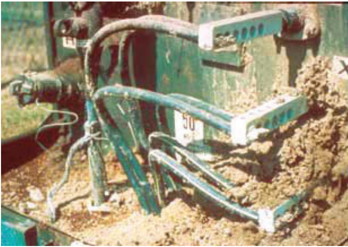
Figure 5. Fire ant mounds in electric utility housing. Credits: S.B. Vinson
